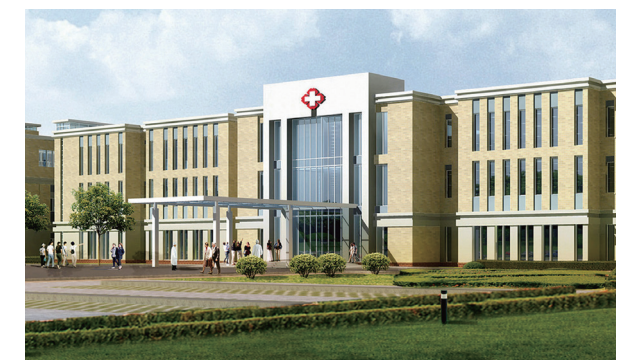
医疗配套——上海市第六人民医院东院 Hospital- Shanghai Sixth People's Hospital Lingang Branch
